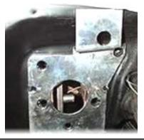
Center punch the marked location to keep the drill bit from wandering. Drill a clearance hole with a 3/8" bit.
